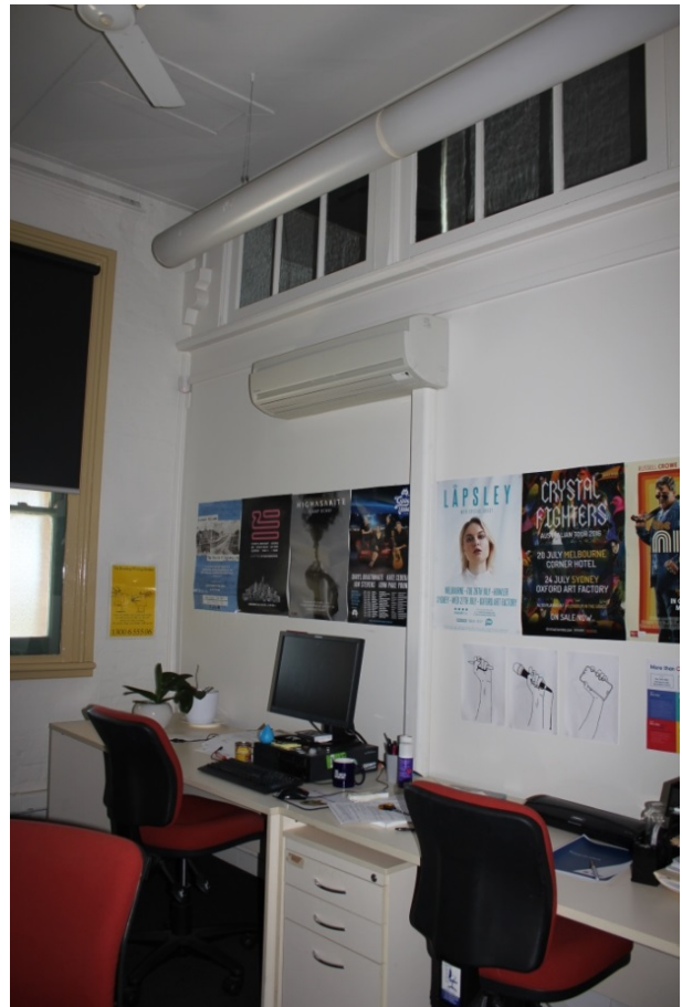
2 Images of the timber-framed glazed partition wall proposed to be removed.
